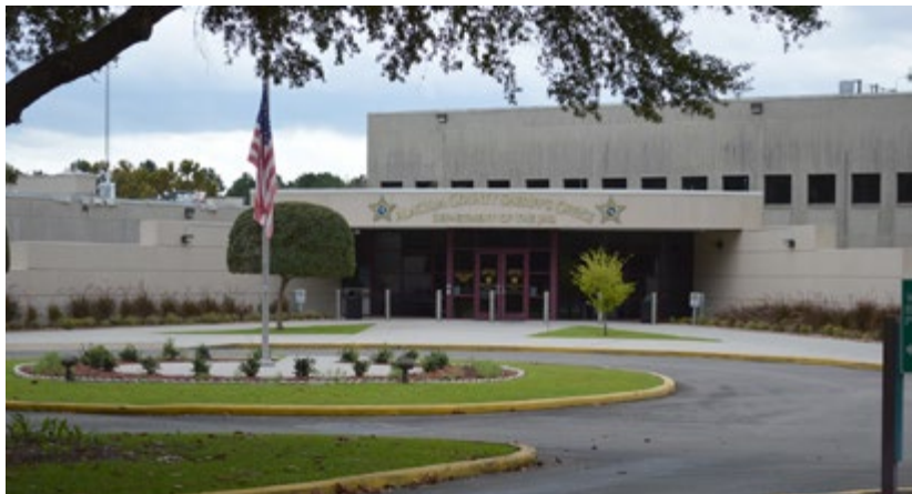
Figure 2. The Alachua County jail has a new chiller plant that is saving electricity compared to when the building was cooled by 78 rooftop air conditioning units.
